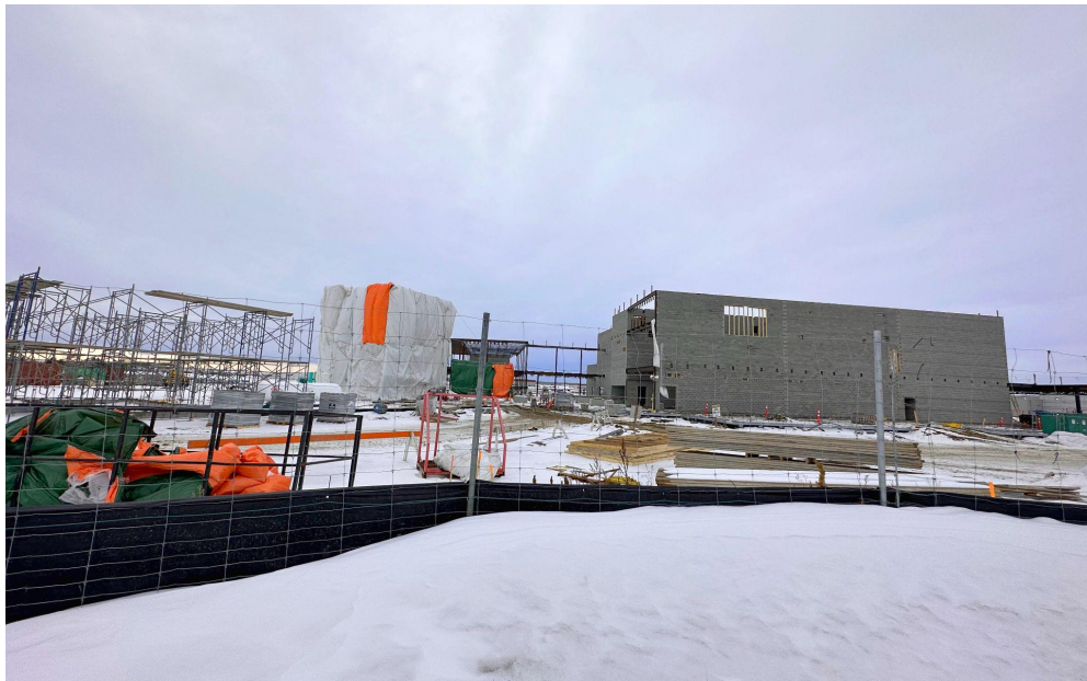
Iron Ridge Secondary Campus - Under Construction February 2023
